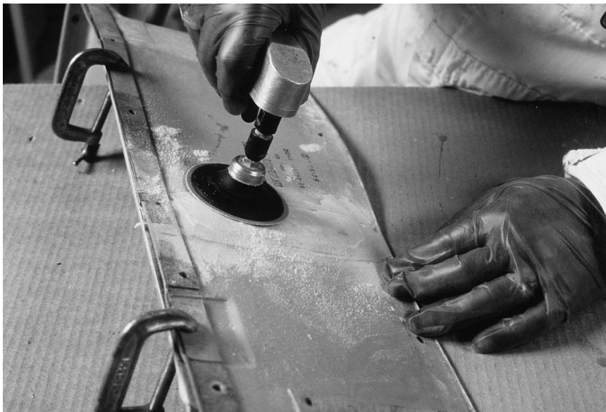
Fig. 7. After curing, the repaired cockpit panel is then sanded and finally painted prior to being reinstalled into the aircraft.
